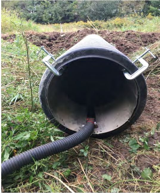
Figure A 19. Close up of area velocity flow probe the outflow of site DY at period when site DY is not spilling.
